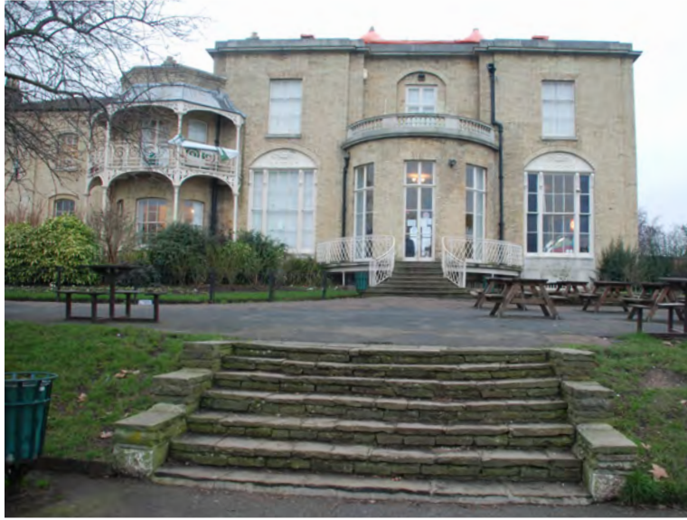
Fig 11.1 (above) Existing Cafe and Terrace
